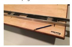
Choose a mounting location for the display and mark the wall center location at the desired height. (Don't forget to account for the
